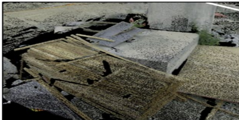
Figure 9. Construction Waste at Pier 27 point cloud initial data
